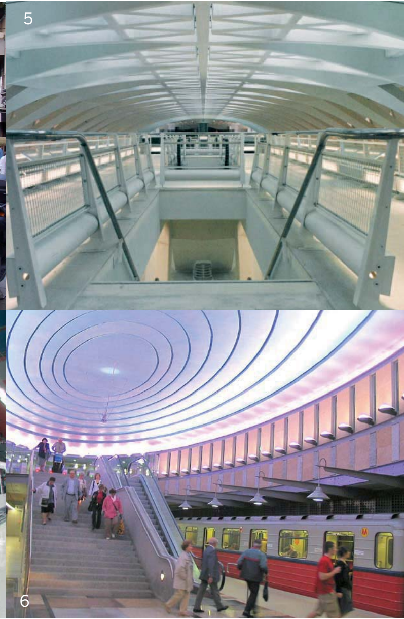
6. Metro de Varsovia, Polonia. 6. Warsaw Metro, Poland.
